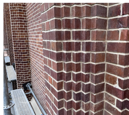
Repointing of deteriorated lime-based mortar to brickwork using new lime mortar, not cement-based mortar.
