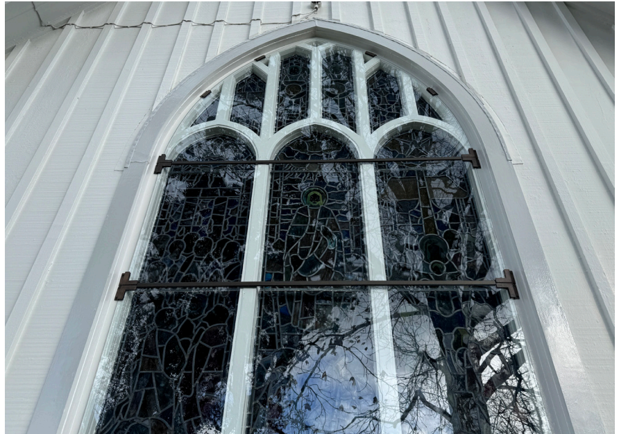
Fabricating and fitting a protective toughened glass screen over a stained glass window using bespoke brackets that can be easily removed for cleaning or in the event of damage to the glass.
