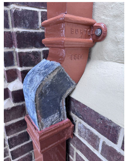
Replacing a broken section of cast iron with lead sheet (to be painted to match), rather than removing and replacing any cast iron.
