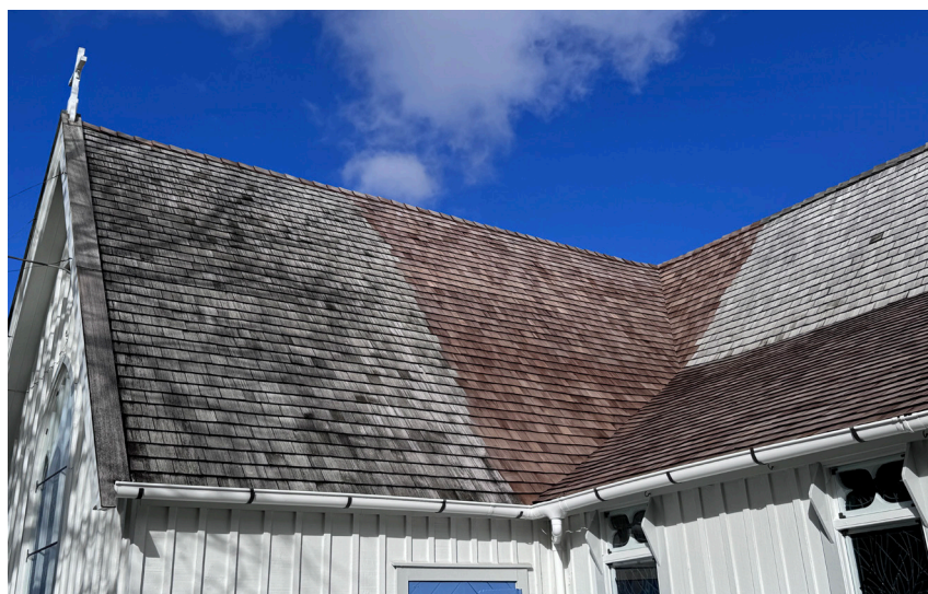
Partial replacement of shingles to eliminate a roof leak, whilst keeping existing shingles that remain fit for purpose, and not artificially treating the new materials to mimic the old.
